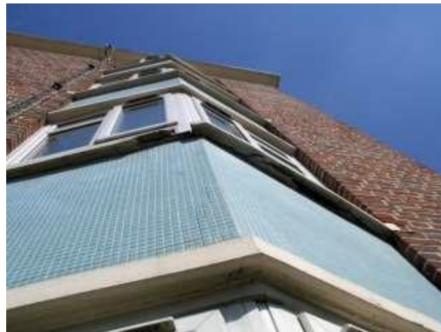
Above and Above Right: Various concrete cills showing cracks and delamination requiring concrete repairs and renewal of window perimeter cills.
