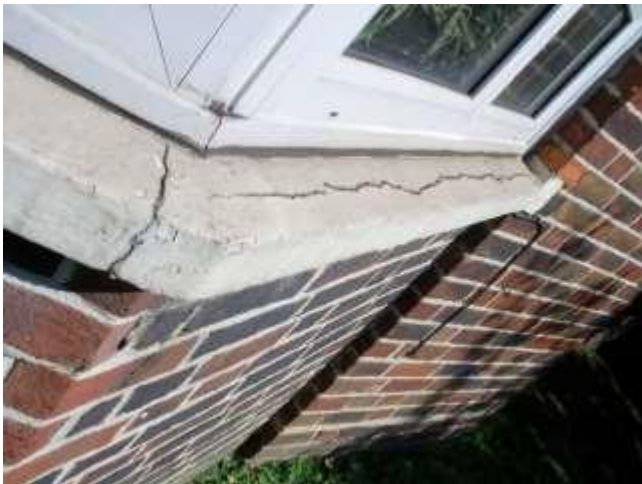
Above and Above Right: Various concrete cills showing cracks and delamination requiring concrete repairs and renewal of window perimeter cills.
